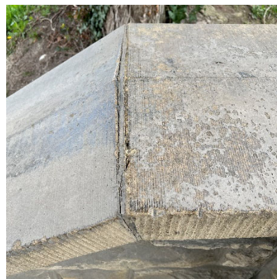
Margelles descellées, joints ouverts, badigeon ciment
